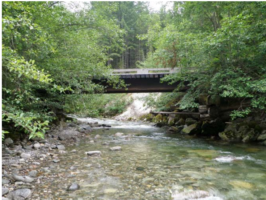
Looking upstream to structure
